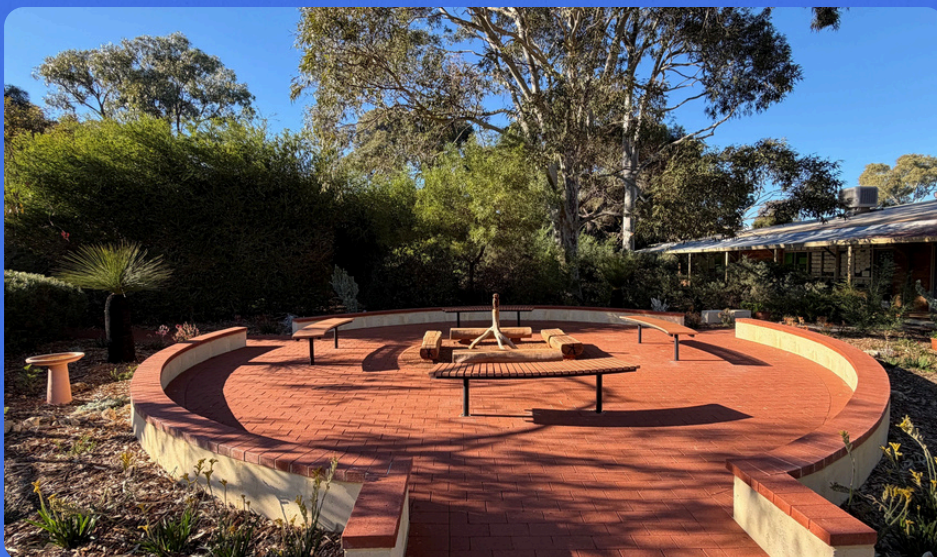
New Yarning Circle/Outdoor Classroom completed!
